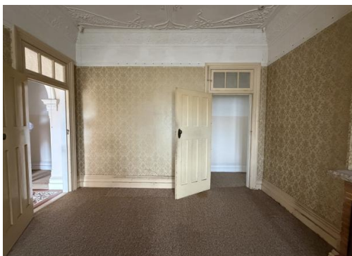
Figure 4.19 Living room showing internal doors with fanlights and decorative plaster ceiling. Wallpaper below timber picture rail.
