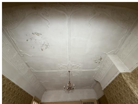
Figure 4.20 Detail of decorative plaster ceiling and cornices. Evidence of water ingress from above.
