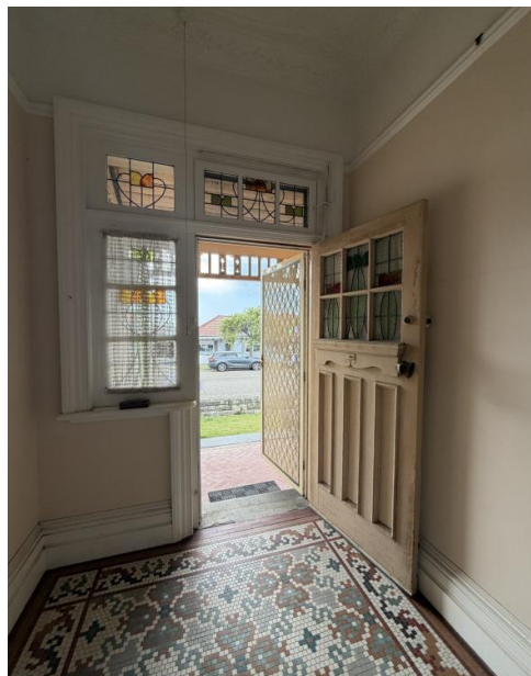
Figure 4.18 Main entry door with fanlights and sidelight and stained glass within upper door panels.
