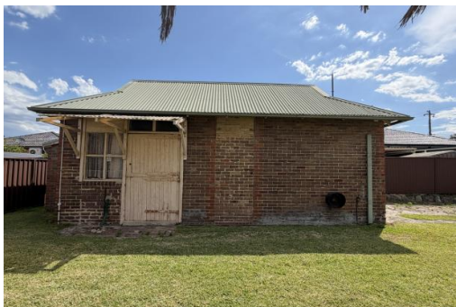
Figure 4.35 East elevation of garage/store showing location of former doorways now bricked in.
