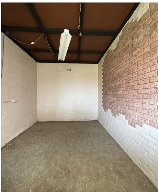
Figure 4.37 Internal view of storage area with brickwork infill.
