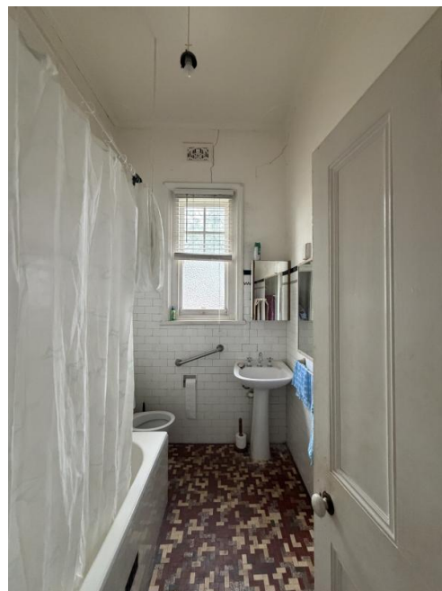
Figure 4.24 View to bathroom with later addition floor and wall finishes and fixtures. Note cracking to northern wall. Undecorated ceiling and original decorative wall vent
