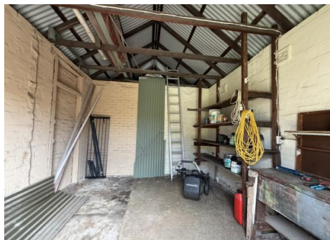
Figure 4.36 Interior of garage/store with decorative vents indicating the space may have been used for accommodation. The flooring is brick paved
