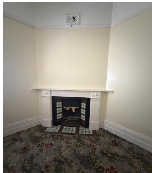
Figure 4.30 Room with fireplace, timber fire surrounds and decorative ceramic tiling and cast-iron grate.
