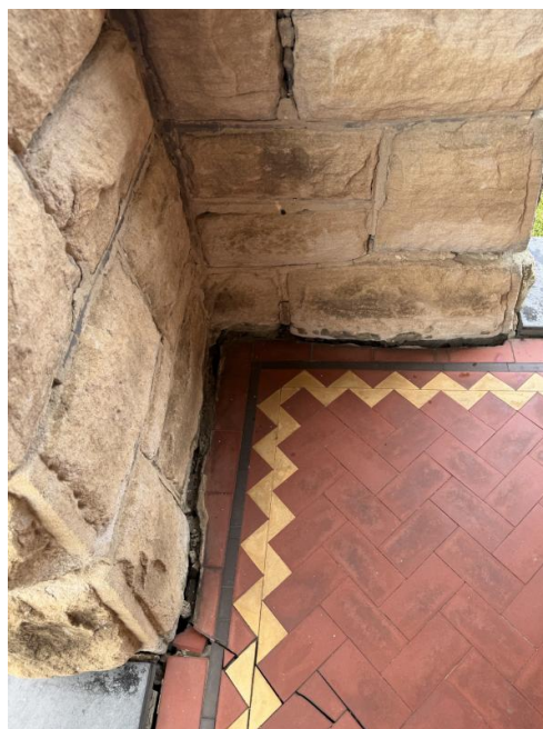
Figure 4.16 Verandah flooring has cracked tiles and structure requires repair works.
