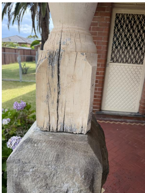
Figure 4.15 Timber verandah post in poor condition.
