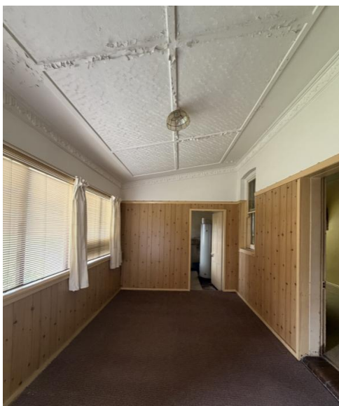
Figure 4.31 Western room is a former deck area has been infilled with view to adjacent laundry. Later addition ceiling, cornices and timber lining.
