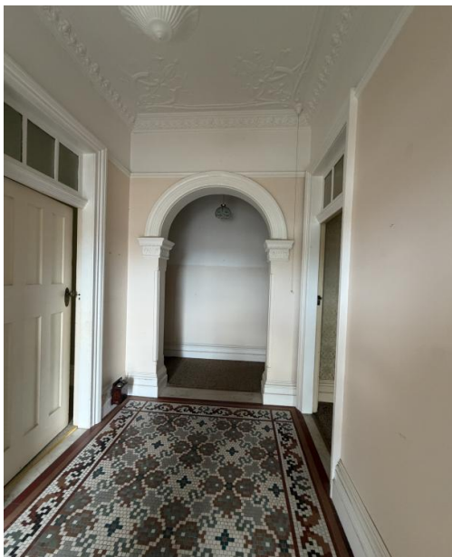
Figure 4.17 Main entry hall showing the arched detail, decorative plaster ceiling, fanlights over doors, and later addition tiled floor.
