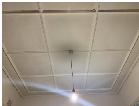
Figure 4.28 Details of decorative plaster ceiling and cornices that are simple in design.
