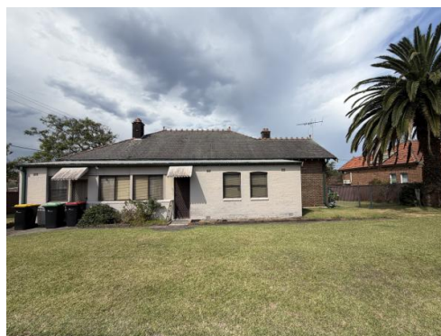
Figure 4.12 View of the west elevation of the residence showing the later addition infilled area between the original two rear wings.
