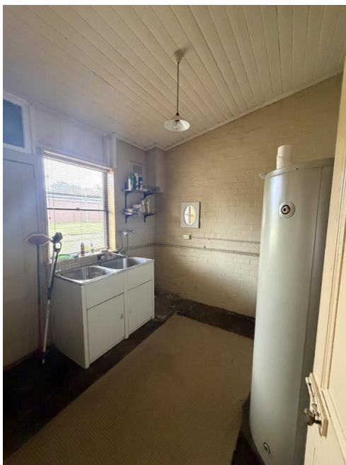
Figure 4.23 Laundry forms part of the original structure with skillion roof lined with timber panelling.
