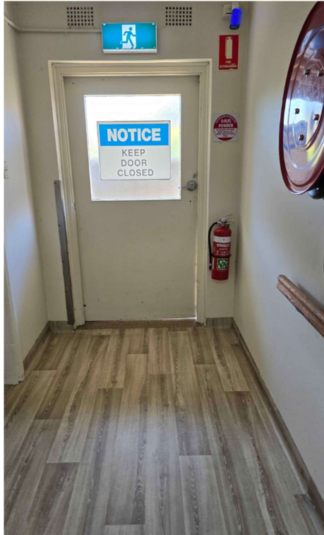
Figure 7: The property has fire safety measures in place including hose reels and fire extinguishers.
