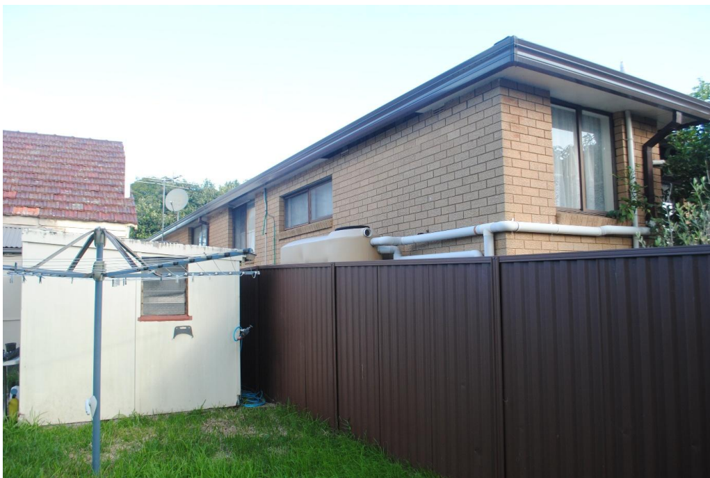
Photo 16 – Rear relationship with No. 16 Hambly Street to the west
