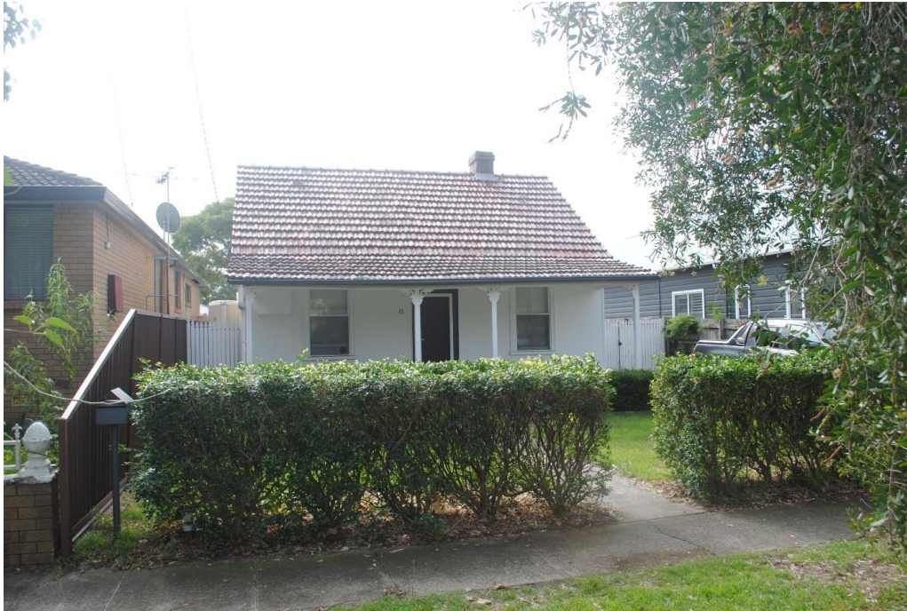
Photo 1 – Subject site and adjoining dwellings
