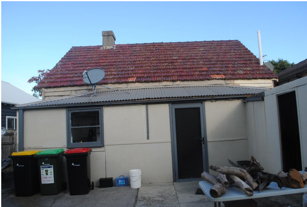
Photo 12 – Existing rear elevation
