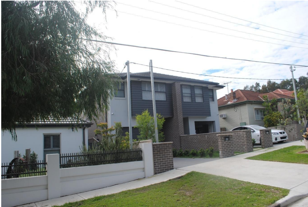
Photo 10 – Nos. 26-28 Hambly Street further east of the site
