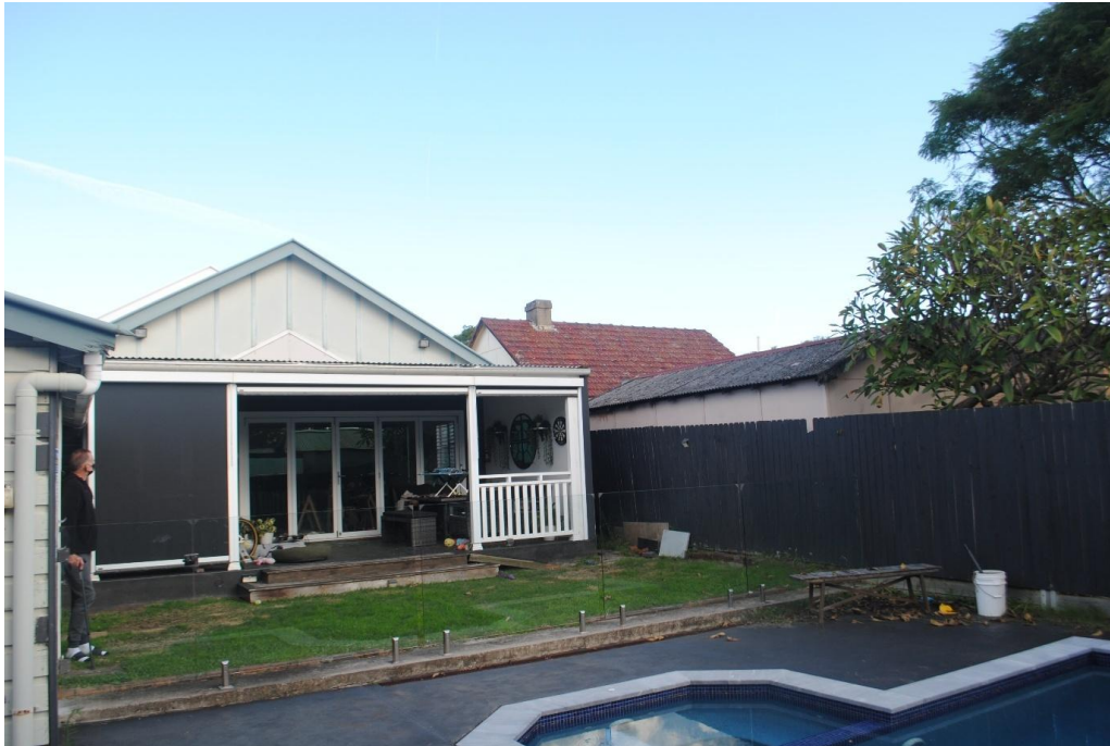
Photo 16 – Rear relationship with site from rear of No. 20 Hambly Street to the east
