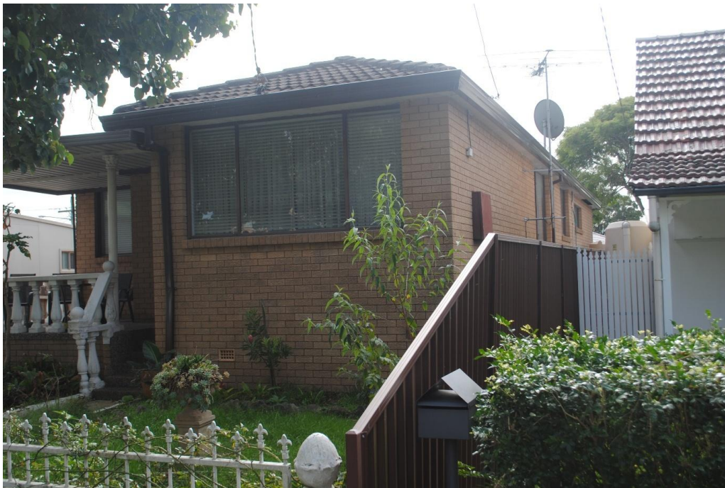
Photo 2 – Adjoining No. 16 Hambly Street to the west
