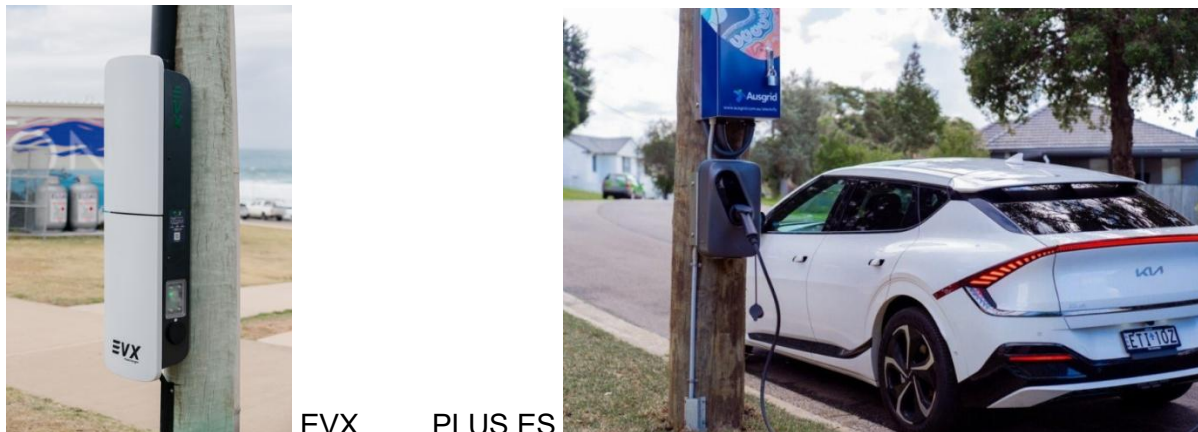
Figure 1: Examples of pole-mounted EV chargers by EVX (left) and Plus ES (right)
