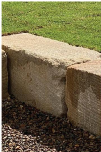
Sandstone log as gravity walls
