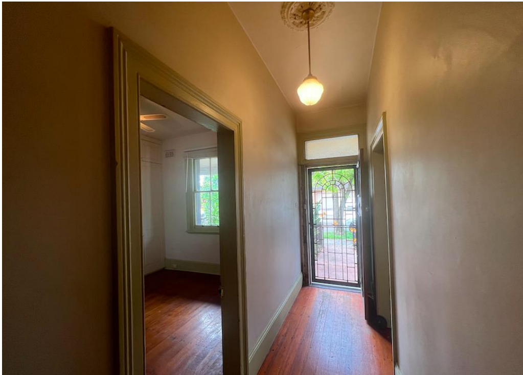
Figure 23 - View of hallway towards front entrance (Source: Three + One Heritage, 2024)
