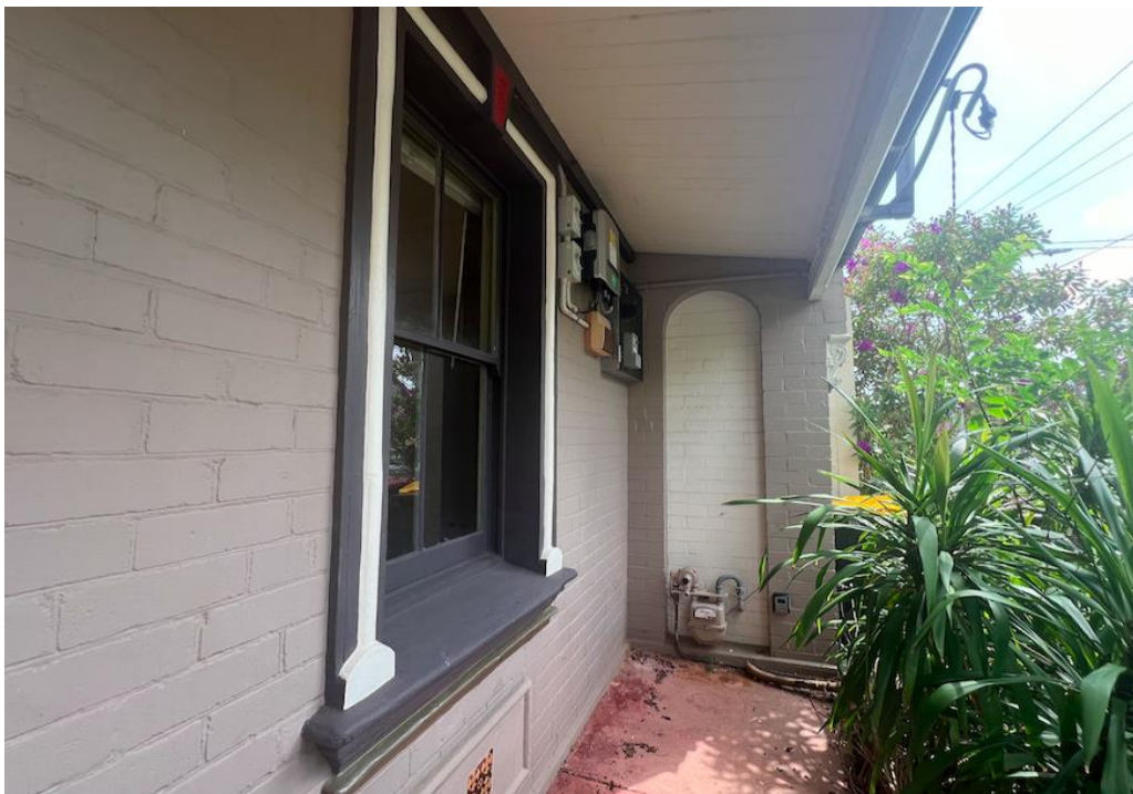
Figure 20 - Front window detailing, view looking north (Source: Three + One Heritage, 2024)
