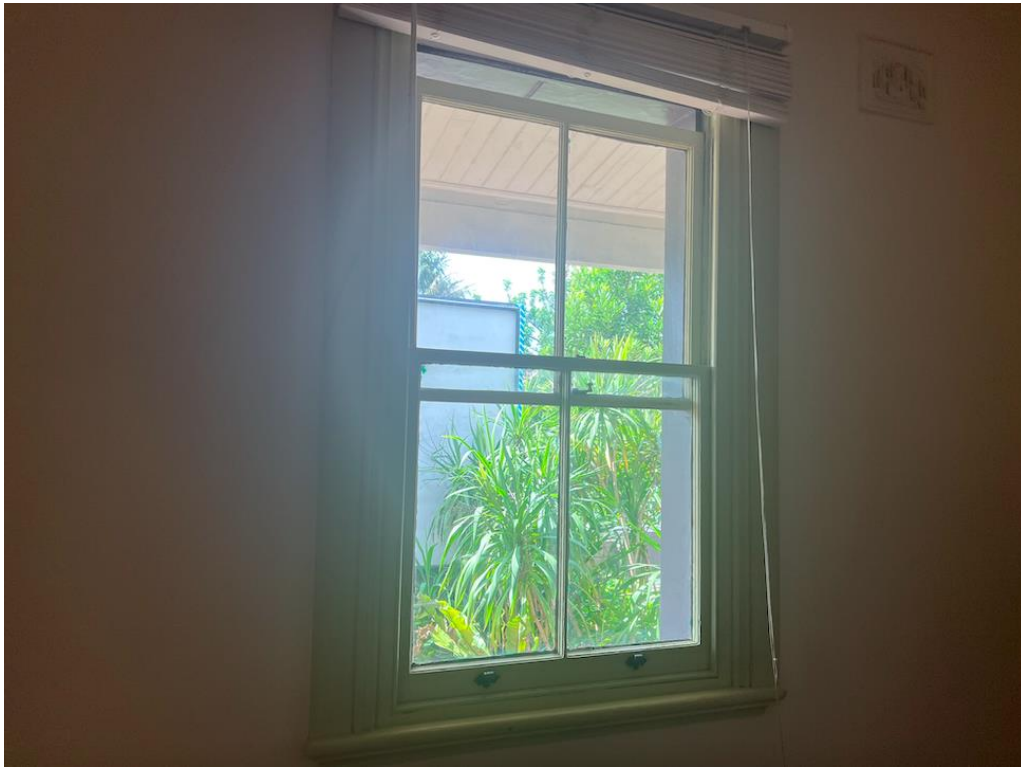
Figure 25 – Timber-framed sash window in Bed 1 (Source: Three + One Heritage, 2024)
