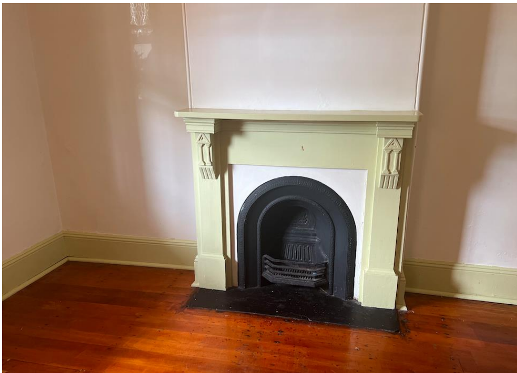
Figure 24 – Existing fireplace in Bed 1 (Source: Three + One Heritage, 2024)
