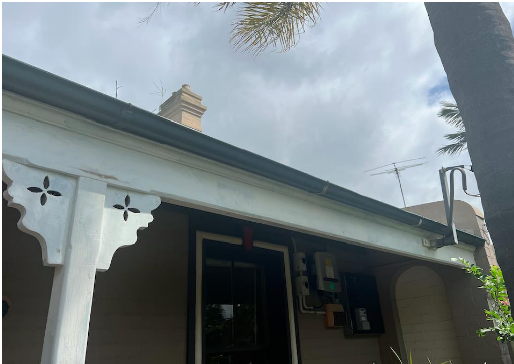
Figure 21 – Timber detailing to the front verandah (Source: Three + One Heritage, 2024)
