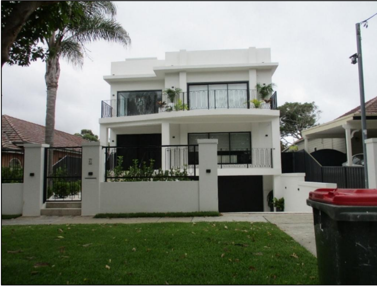
Figure 8: Existing two storey dwelling (No.43) as viewed from Monterey Street
