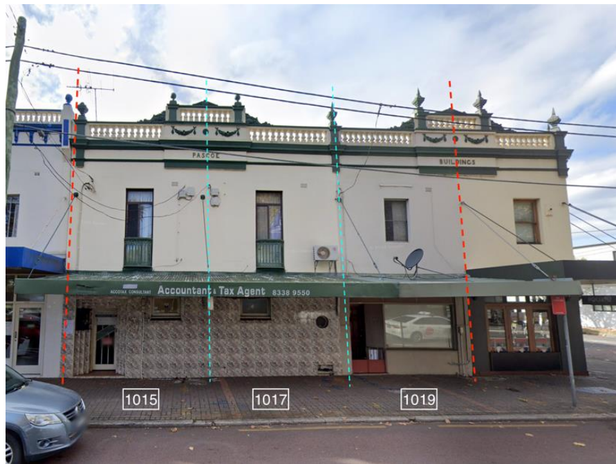
Figure 3: The primary elevation of the site showing the division of the terraces.
