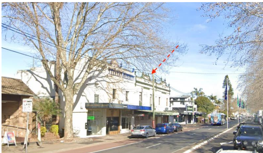
Figure 32: View looking north along Botany Road towards the site.
