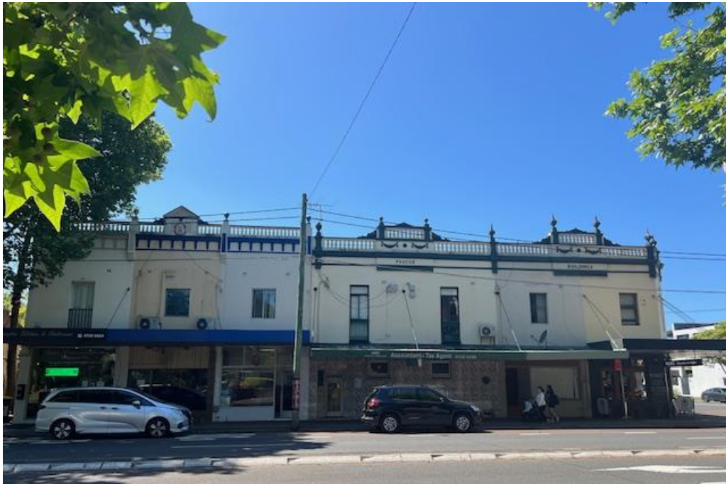
Figure 7. Existing streetscape (No. 1009-1021 Botany Road)
