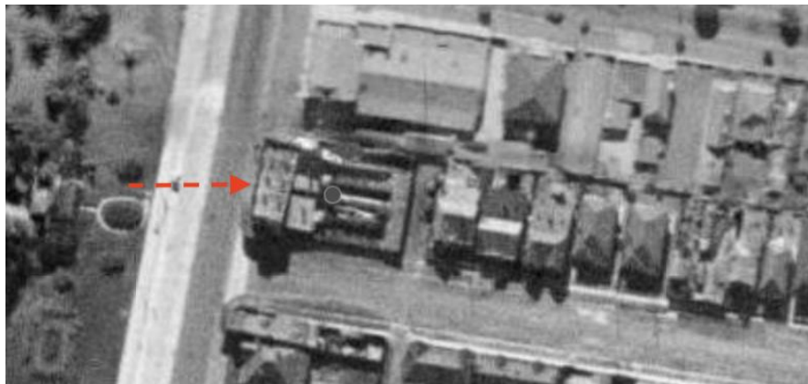
Figure 26: The site in 1943 showing the site and surrounding development.
