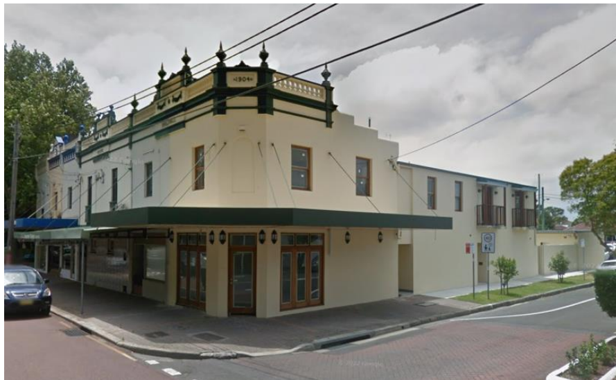
Figure 29: The site in 2015 showing the newly completed addition and repainted façade. Google Maps 2015
