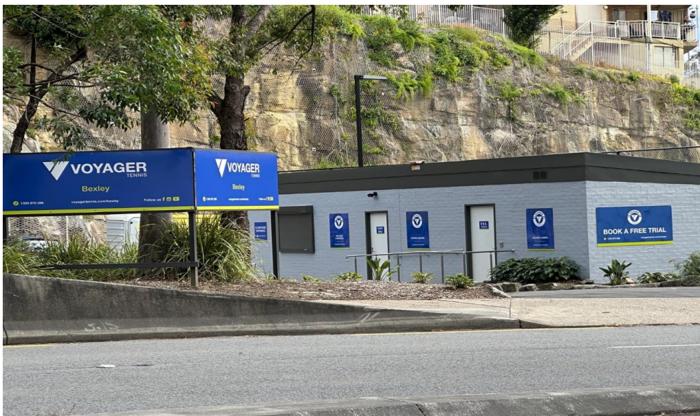
Figure 13. The existing clubhouse building and signage viewed from Bexley Road
