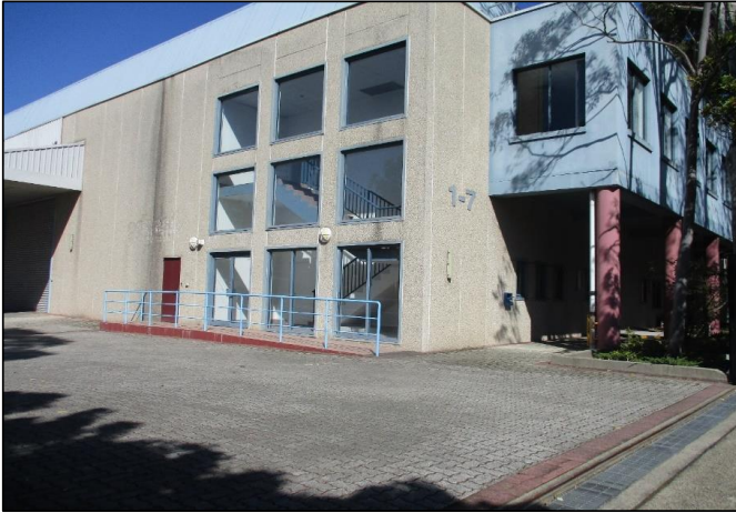
Figure 10: Existing entry ramp to be replaced at 1-7 Green Street, Banksmeadow
