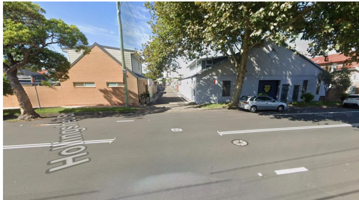
Plate 1: Adjoining 2-storey structure immediately to the north and that immediately opposite
