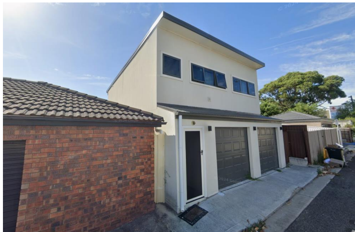
Plate 3: 2-storey structure at 84 Hardie Lane
