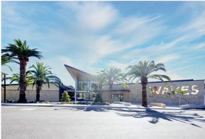
WAVES AQUATIC & LEISURE CENTRE Client – The Hills Shire Council
