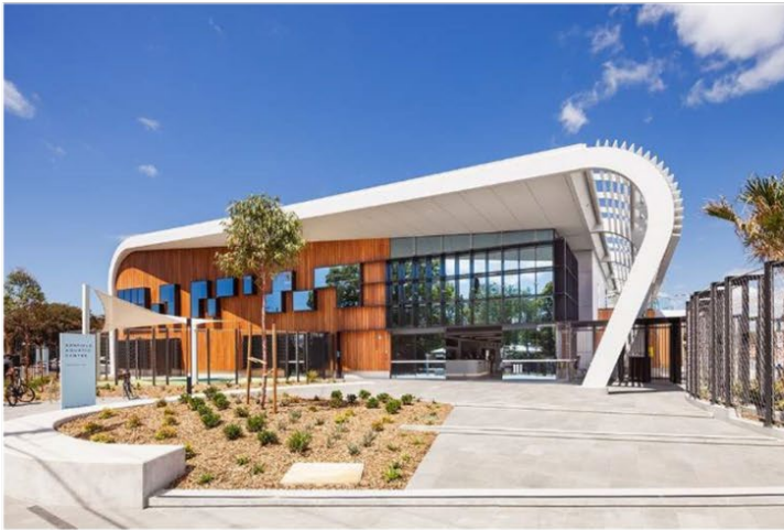
ASHFIELD AQUATIC CENTRE Client – Inner West Council
