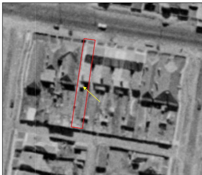
Figure 4. 1955 aerial image of the site, which is outlined in red. Note the addition to the rear of the building indicated by the yellow arrow (Source: NSW Spatial Services, Historical Imagery Viewer, accessed 11 December 2023, annotated by Heritage 21).
