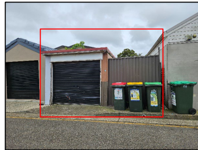
Figure 9. External view to the rear elevation of the subject site, facing south on King Lane.
