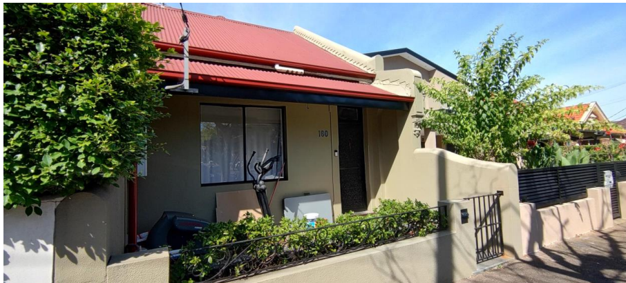
Figure 7 Subject site as seen from King Street
