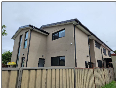
Figure 14. External view to the rear portion of 162 King Street, located to the west of the subject site, facing north-west from within the site.
