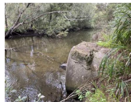
Damaged concrete inlet pipe empties directly into southern Scarborough Pond
