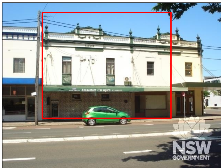
Figure 18: Picture from 2015, showing the subject site No. 1015, 1017, and 1019 Botany Road. Source: NSW State Heritage Inventory, https://www.hms.heritage.nsw.gov.au/App/Item/ViewItem?itemId=1210033 , Accessed April 2022.
