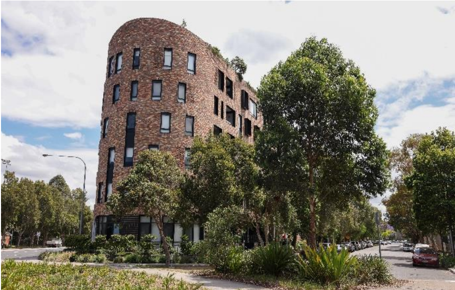
Figure 4: Residential flat building on Huntley Street, Alexandria
