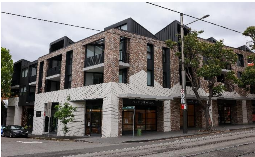
Figure 4: Shop top housing in Surry Hills
