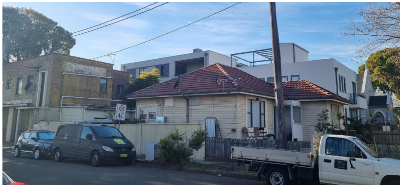
Figure 8: View of the subject site from Tenterden Rd
